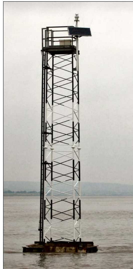
New tower completed
